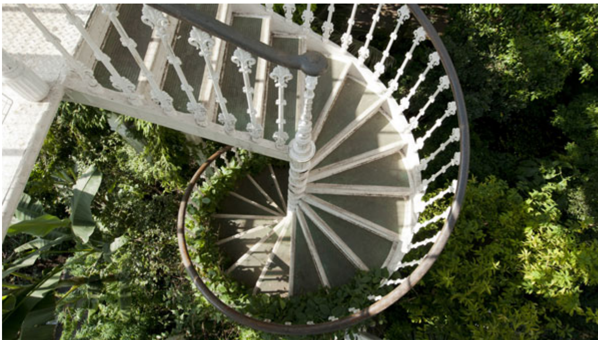
A five year restoration project on the Temperate House at Kew Gardens is almost complete.
