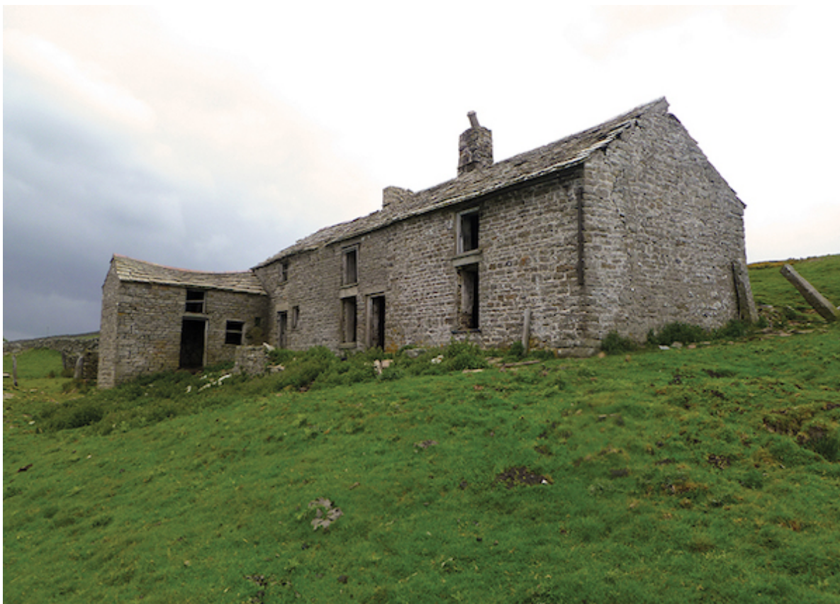
Spain's Field Farm, photographed at its original site in Weardale before being moved brick by brick to Beamish. Courtesy of Beamish
